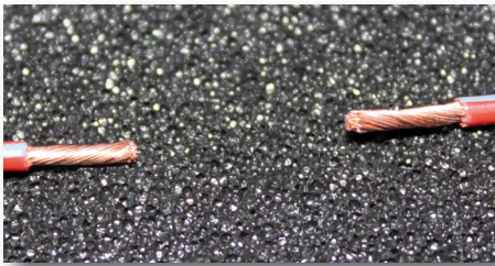
Fig 3.1.4a - Strip and twist the wire ends as described in 3.1.1.
